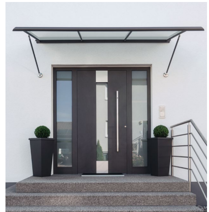
Final result after installation
